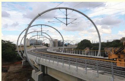
SGR infrastructure in Dar es salaam
